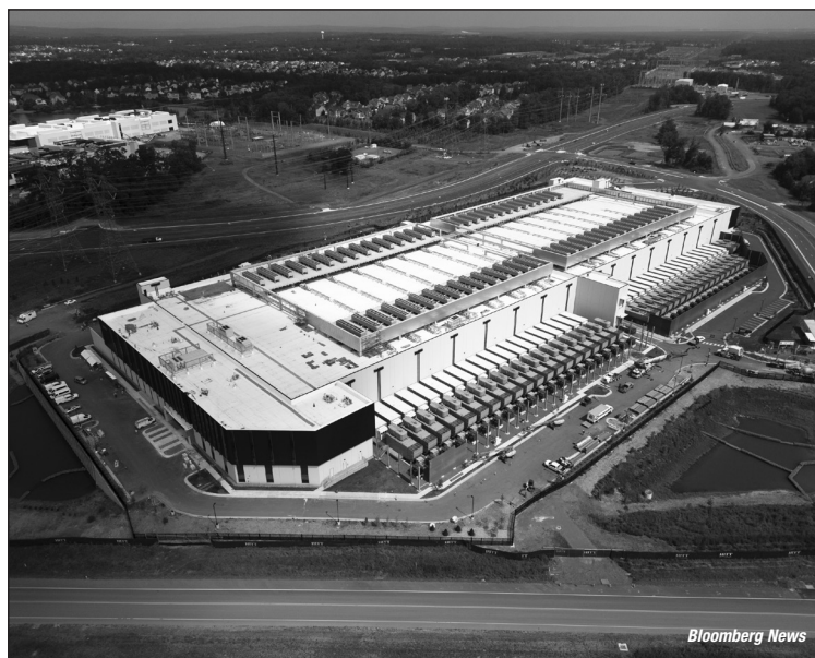
A data center in Virginia. Many data center projects take advantage of tax breaks that can be costly for states and local governments.
